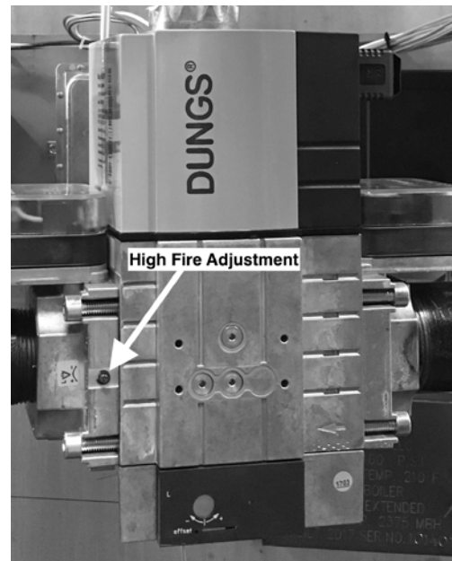
Figure 7: High Fire Adjustment on the Main Gas Valve Regulator (This valve applies ONLY to ARC1000 through ARC3000)
